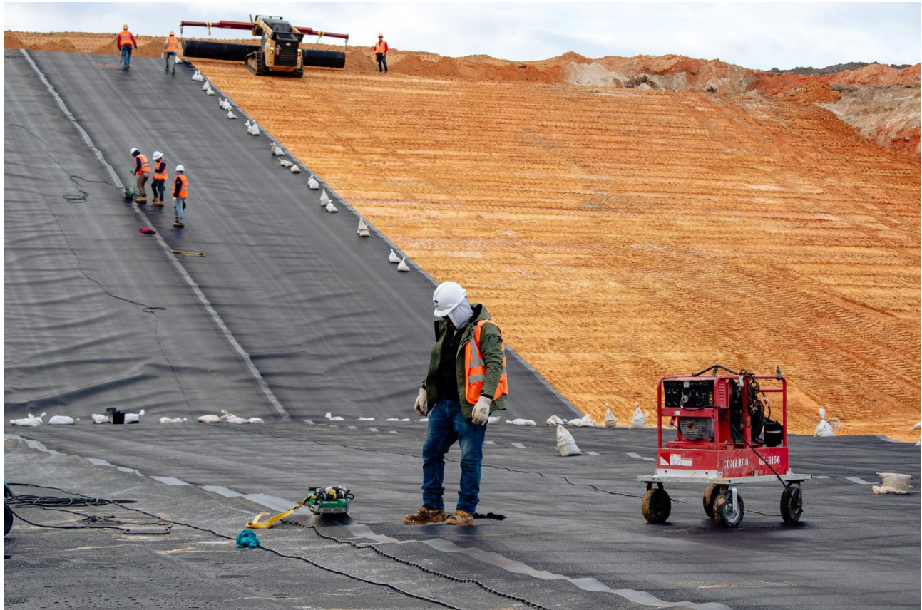
Photo of HDPE liner being installed courtesy of Comanco
